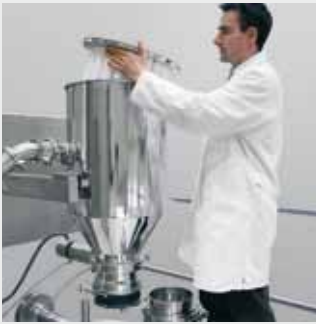
Excellent access to all plant components is shown here for the vacuum conveyor to discharge the dryer.
